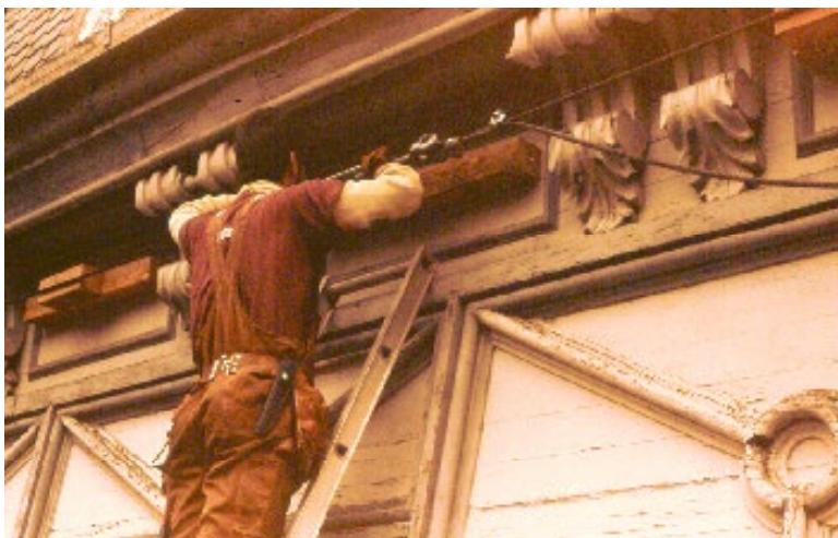
Installation of exterior tension cable & turnbuckles
